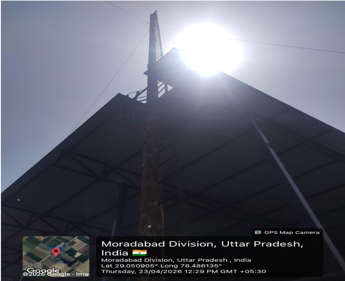
Excess pyro gas flared through stack minimum height of 30 meter
